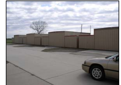
Building Number 6 T-Hangars
