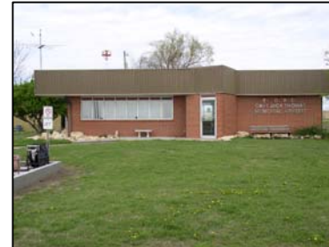
Building Number 2 Terminal Building
