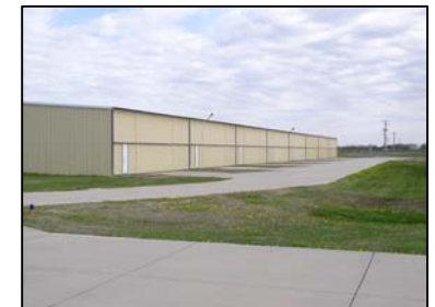
Building Number 7 T-Hangars
