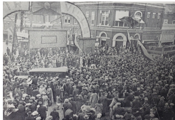
Intersection of Central & Main.
