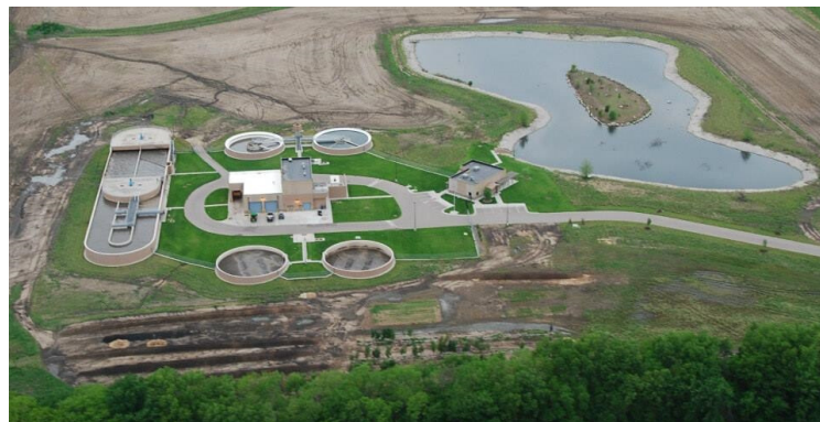
Wastewater Plant Pictures courtesy of Kurt Bookout
