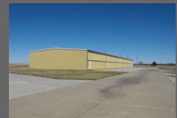
Building No. 8 10 Unit T-Hangars
