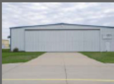
Building No. 5 Conventional Hangar Peterson's Performance Plus
