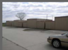
Building No. 6 4 Individual T-Hangars
