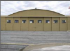
Building No. 4 Conventional Hangar
