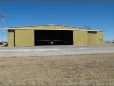
Building No. 3 Conventional Hangar
