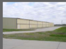
Building No. 7 15 Unit T-Hangars
