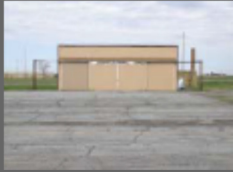
Building No. 1 Conventional Hangar
